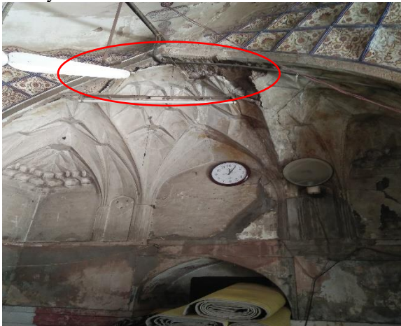
Fig 24: Crack on muqarnas of rightmost bay
