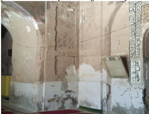
Fig 26: Fresco work vanished and lime exposed
