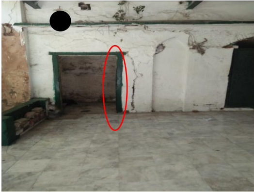
Fig 18: Crack just beside the right side entrance
