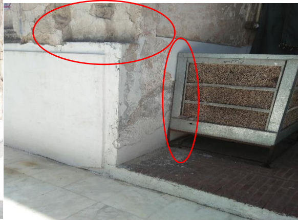
Fig 35: Some major and minor cracks on pillars of bays
