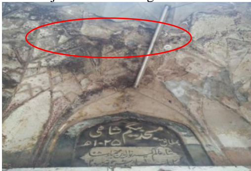
Fig 20: Cracks on main entrance filled with lime
