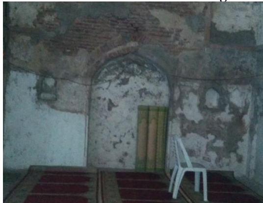
Fig 30: Crack on the left bay wall and fresco work vanishes (self-documented)
