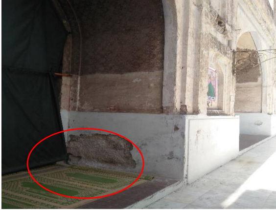
Fig 34: Crack on the column of 2 nd left bay pillars of bays
