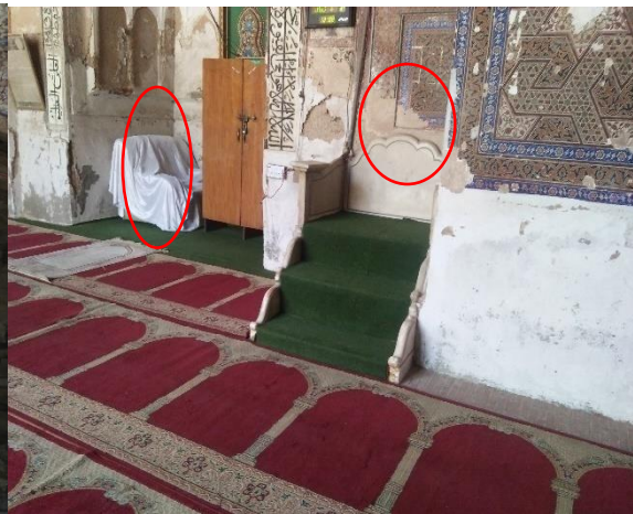
Fig 25: Cracks on the wall beside mehrab roof
