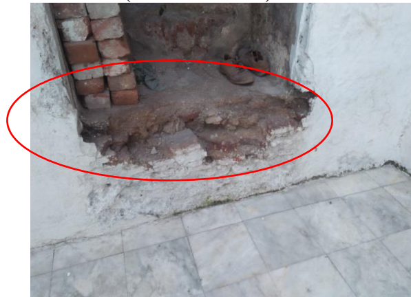
Fig 32: Crack on stairs on left side accessing minarets and domes
