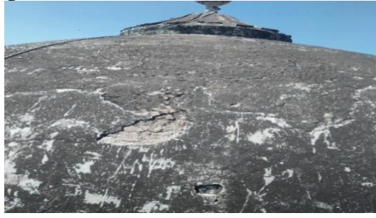
Fig 42: Cracks on exterior of domes
