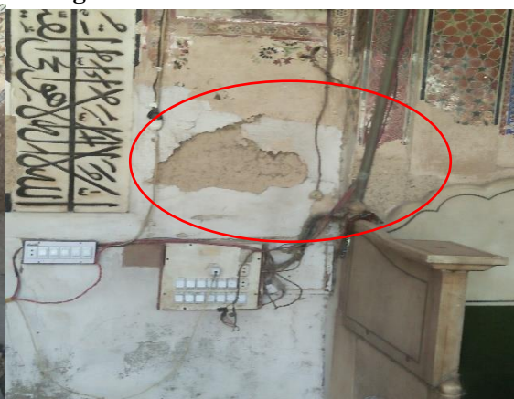
Fig 27: Material deteriorated from wall mortar is being exposed
