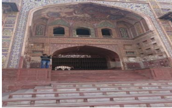
Fig 13: Light striking the facade
