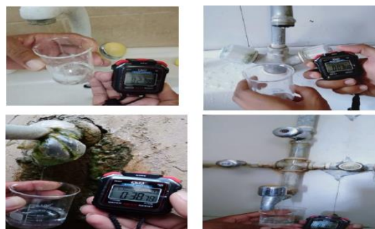
Fig.2 Measurement of leaks at various places
